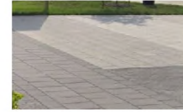
1. PRECAST PAVING BANDS TO MATCH EXISTING
