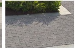
2. EXISTING PERMEABLE PAVERS
